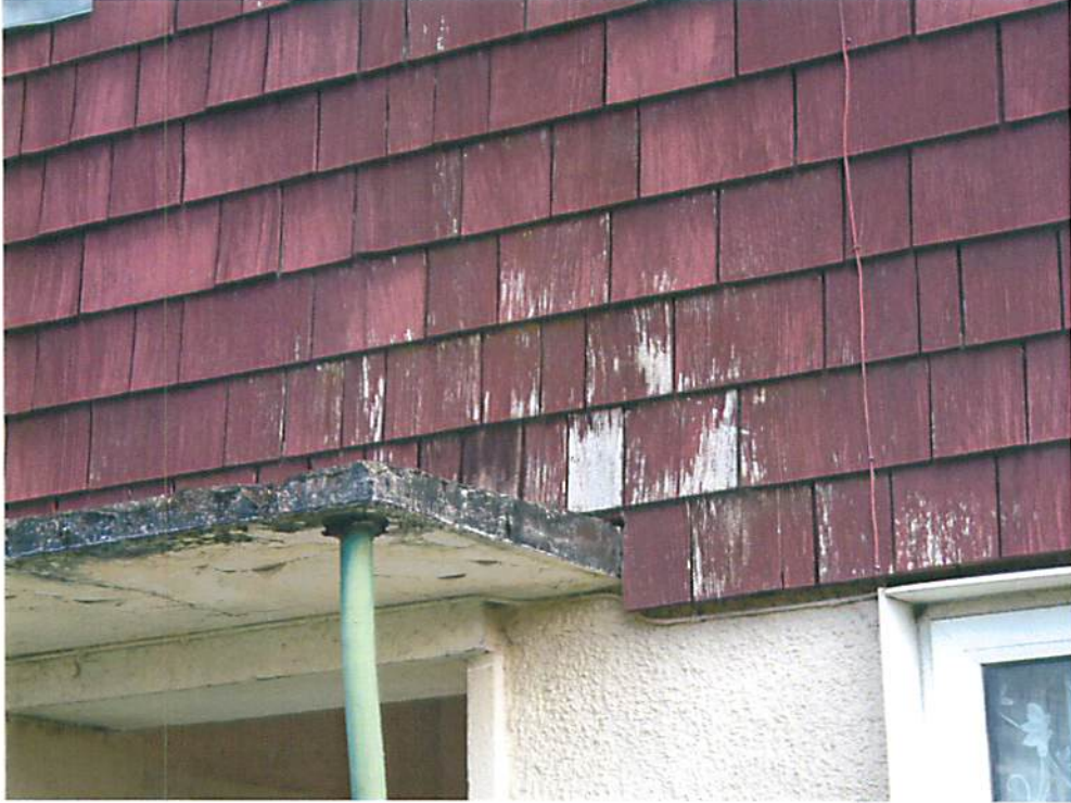
Shingles to front elevation
